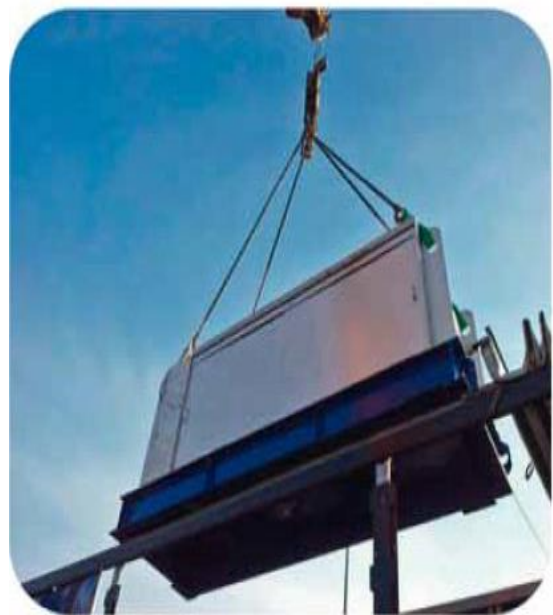
Unloading from the truck, to the hall for installation
