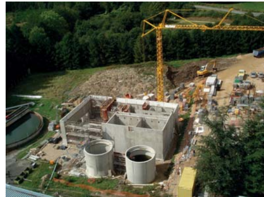
FIG. 2, INDUSTRIAL PLANT VERTOLAYE (F), DURING CONSTRUCTION
