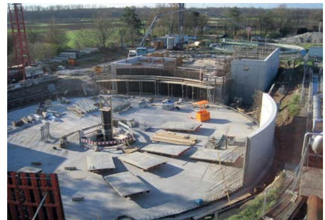
FIG. 3, WWTP LAHR (D), DURING CONSTRUCTION
